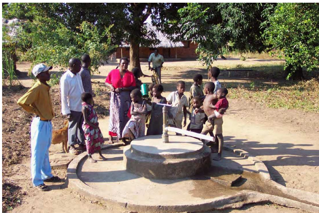
Plate 75 Mark V pump on a shallow well
