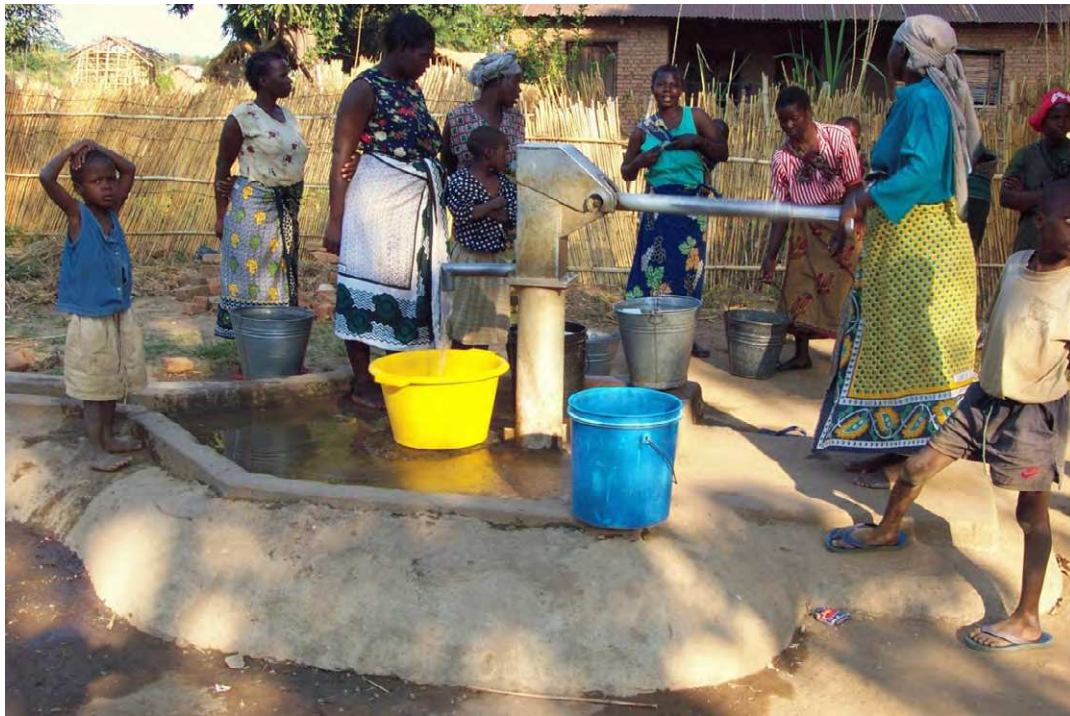
Plate 72 Afridev pump on borehole
