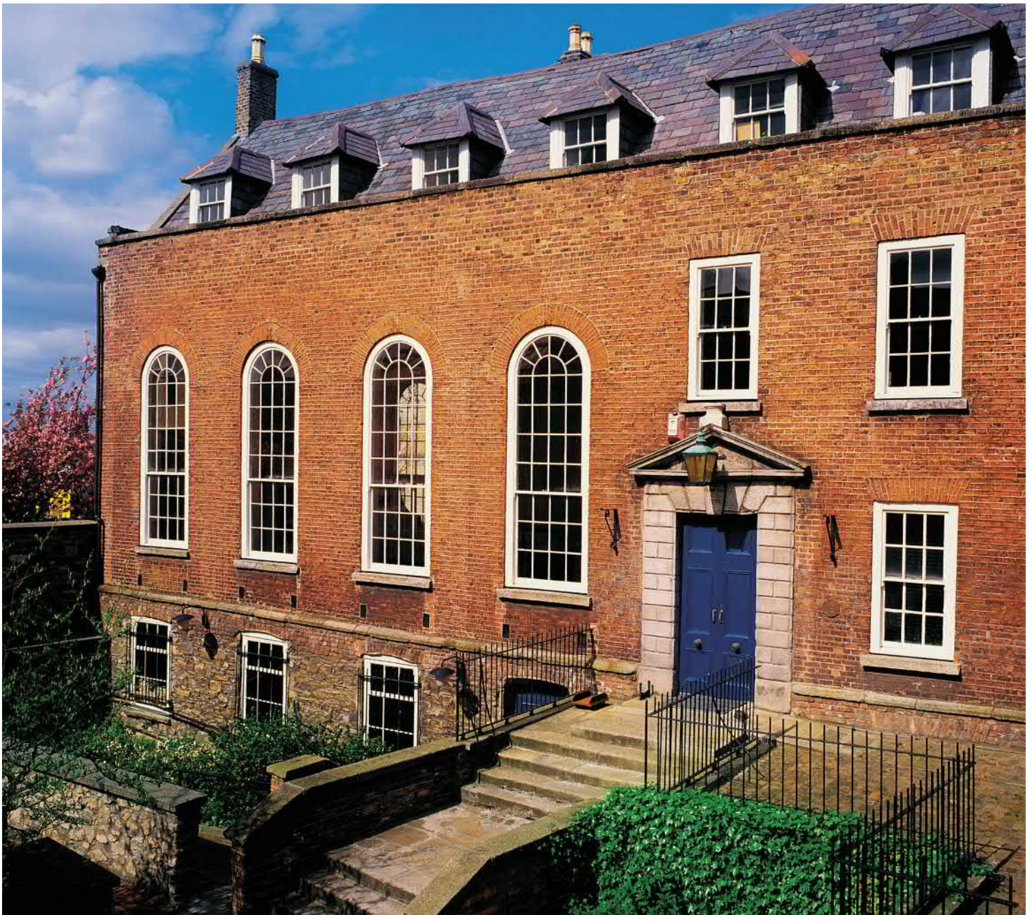
▲ The red-brick façade of Tailors' Hall, restored to its former glory
