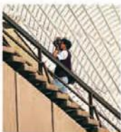
Opera House roof tiles
