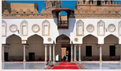
Arcaded courtyard of the Mosque of al-Azhar, Cairo
