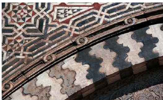
“Joggling” on southern facing arch of Sabil-Kuttab of Abdel Katkhuda
