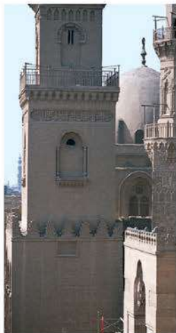
View across the rooftops to the balconies on the minaret of the Madrasa of Sultan Barquq
