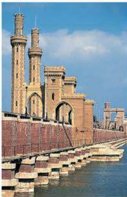
Nile Barrages at Qanater, where the two branches of the river fork
