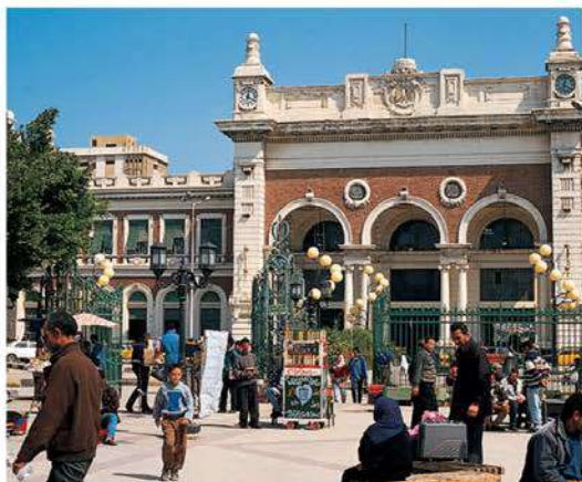
Façade of the Masr train station in central Alexandria
