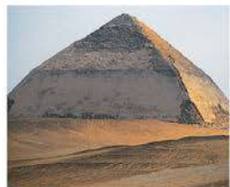
Sneferu's Bent Pyramid at Dahshur with much of its outer limestone casing still visible
