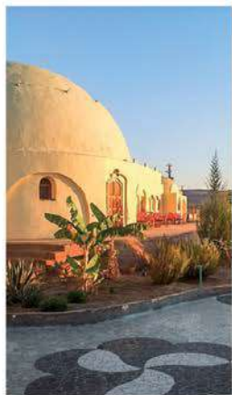
One of the domed accommodation buildings at the Bawiti Oasis Resort (see p277)
