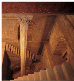
Nilometer on Rhoda Island showing the simple calibration used to predict the floods
