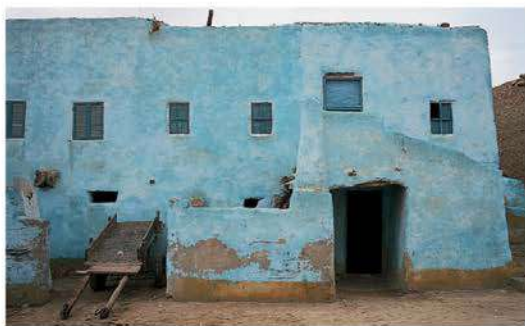
A blue-painted mudbrick dwelling in Siwa Oasis
