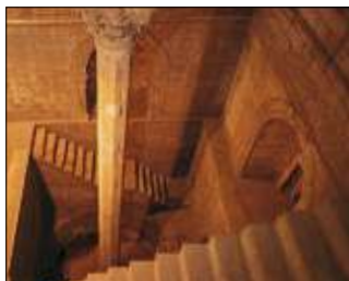
Nilometer on Rhoda Island showing the simple calibration used to predict the floods
