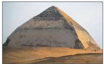
Sneferu’s Bent Pyramid at Dahshur with much of its outer limestone casing still visible
