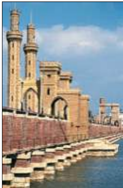
Nile Barrages at Qanater, where the two branches of the river fork
