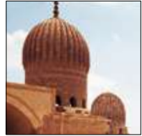
The dome of Madrasa Sultaniya (c.1370) in the City of the Dead (see p103) has a rib design.
