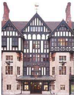
Liberty's mock-Tudor façade
