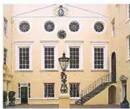
Apothecaries' Hall, rebuilt in 1670
