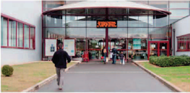
Entrance to the Centre Aquatique Nautilus in St-Yrieix-sur-Charente
