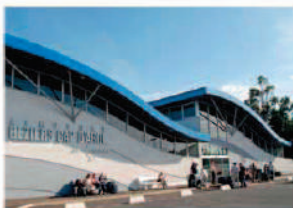
Wave-like roof of Béziers Cap d'Agde airport, close to the Languedoc beaches
