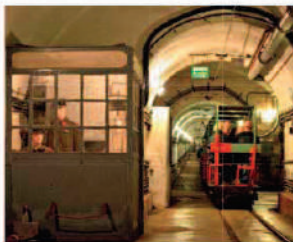
A train chugging through a tunnel of one of the forts of the Maginot Line
