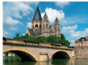
One of the 20 bridges spanning the river in Metz
