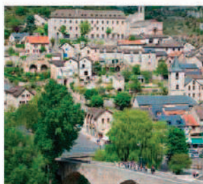
The Ste-Enimie bridge and a grand view of the town
