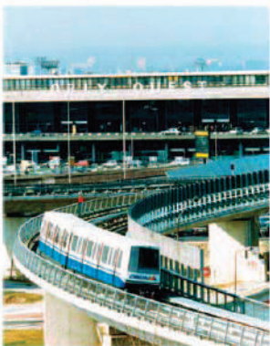
The Orlyval train connecting Orly Airport to the metro system
