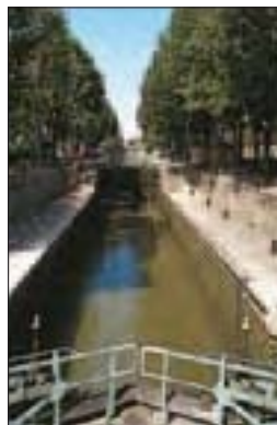
View from Rue E Varlin bridge ⑦
