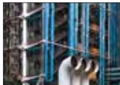
Pompidou Centre See pp110–13.
