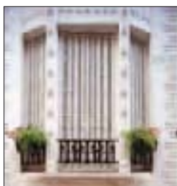
Shuttered bay window at No. 3 Square Jasmin ⑬
