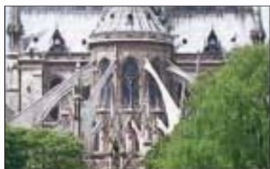
★ Flying Buttresses Jean Ravy's spectacular flying buttresses at the east end of the cathedral have a span of 50 ft (15 m).
