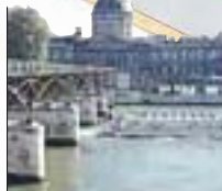
The Passerelle des Arts is a steel reconstruction of Paris's first cast-iron bridge (1804), and was inaugurated in 1984.
