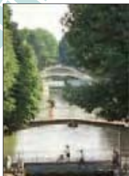
Iron footbridges over the canal ⑬
