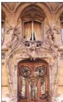
Doorway at No. 29 Avenue Rapp
