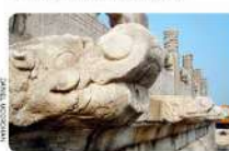
Dragon-Head Spouts More than a thousand dragon-head spouts enliven the raised marble platforms at the centre of the Forbidden City. They were – and still are – part of the drainage system.
