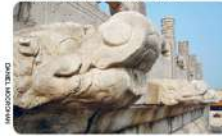
Dragon-Head Spouts More than a thousand dragon-head spouts encircle the raised marble platforms at the centre of the Forbidden City. They were – and still are – part of the drainage system.
