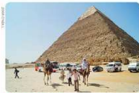
Pyramid of Khafre Khufu's son built this pyramid, which has some surviving limestone casing at the top. Scattered around the base are enormous granite stones that once added a snappy black stripe to the lowest level of the structure.
