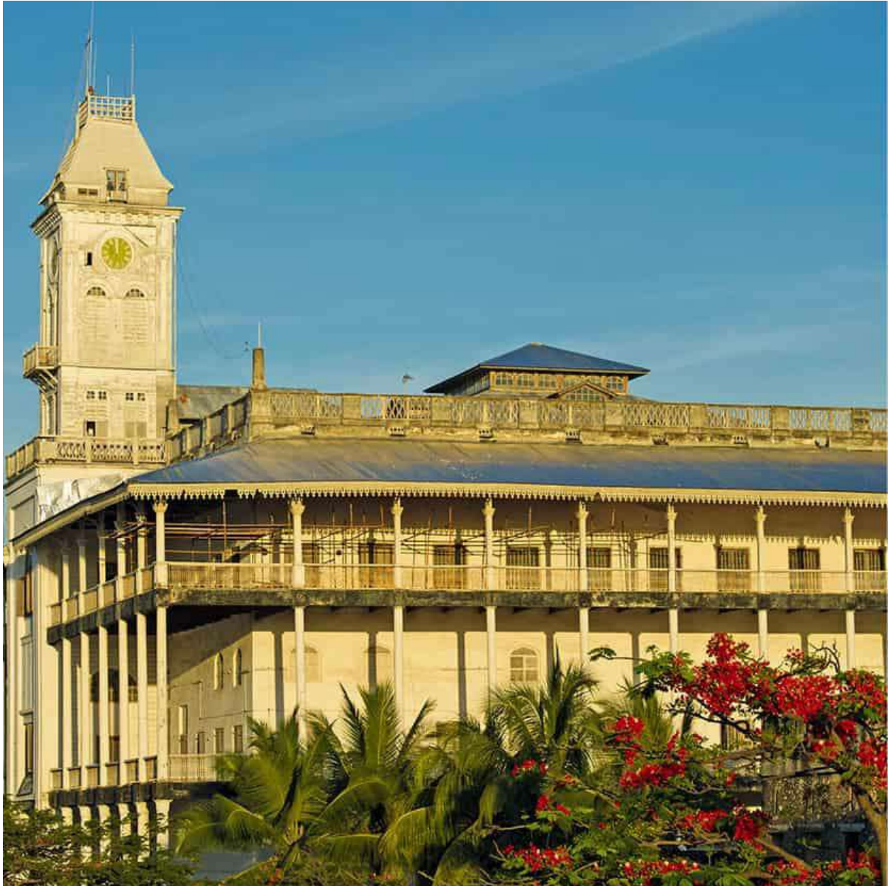
The House of Wonders, one of Stone Town's most impressive buildings. Ariadne Van Zandbergen/Apa Publications
