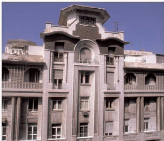
The Glaoui residential block, built in 1922 by M. Boyer
