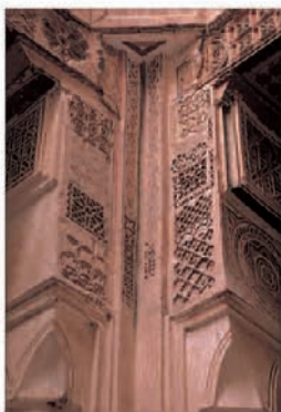
Detail of the interior of the ksar at Tamnougalt, in the Draa valley
