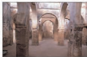
The interior of the mosque built by Abou Youssef
