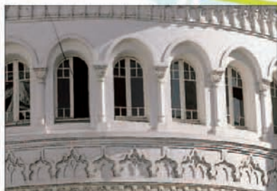
Detail of a 1930s façade in Casablanca
