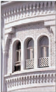
1930s architecture features traditional Moorish elements, including semicircular arches and decoration in the form of carved stucco.
