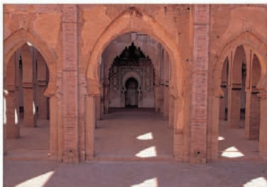
The mosque at Tin Mal, with pink brickwork and plaster stalactites
