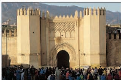
The monumental gateway, a fortified entrance flanked by projecting crenellated towers, leads into the medina. Bab el-Cborja in Fès is a particularly splendid example.
