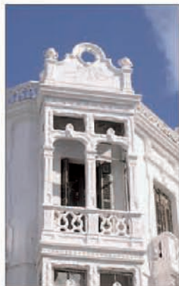
Detail of a façade on Boulevard Mohammed V
