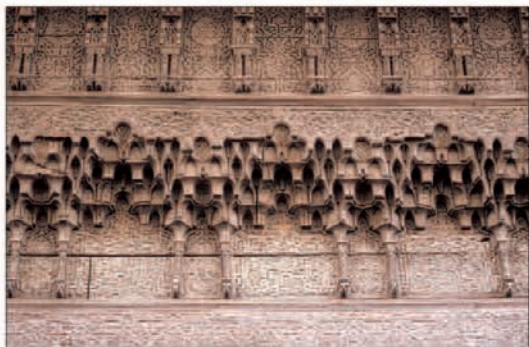
Detail of the cedar awning over the Chrob ou Chouf Fountain
