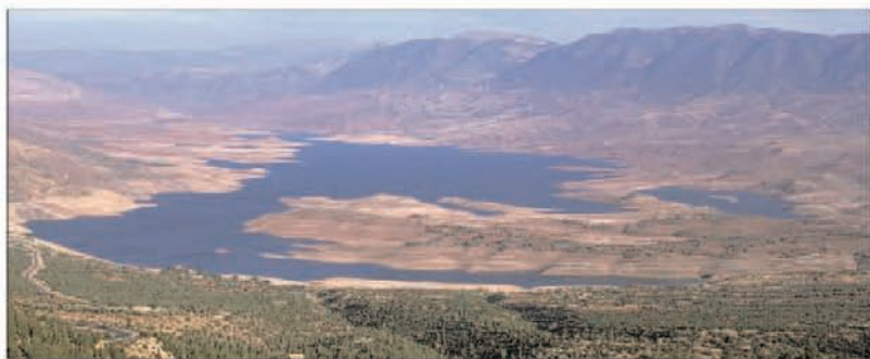
The Bin el-Ouidane reservoir, at the foot of the High Atlas
