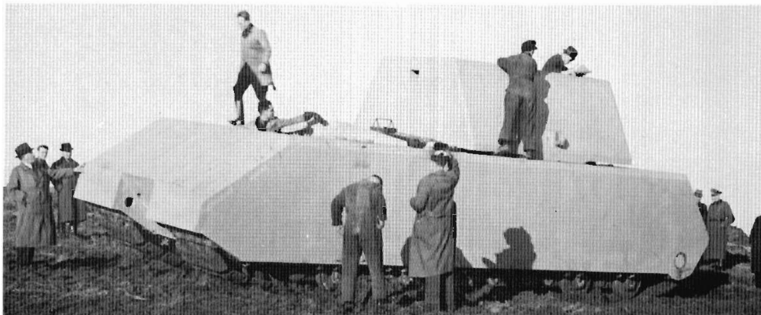
Plate 494. Pz Kpfw 'Maus' prototype on trials, with simulated turret. (See also Plate 27, Page 12.)
