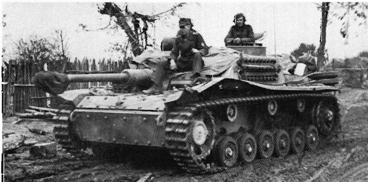
Plates 257-259. StuG III Ausf G. (Note, in Plate 259, the additional armour bolted to the front of the vehicle.) Plate 260 (opposite page, top). StuG III Ausf G with Saukopf gun mantlet.
